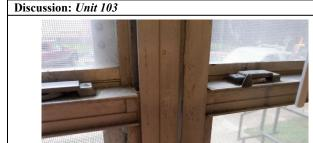
Sealant Visible at Mulled Window Unit
